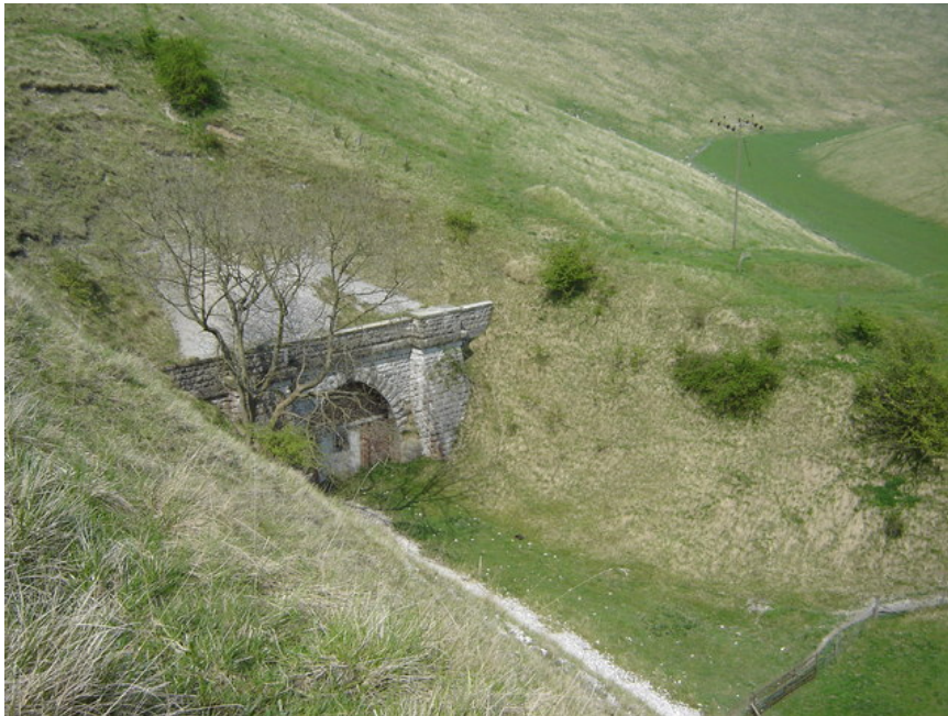
Burdale tunnel entrance, the only entrance visible.
