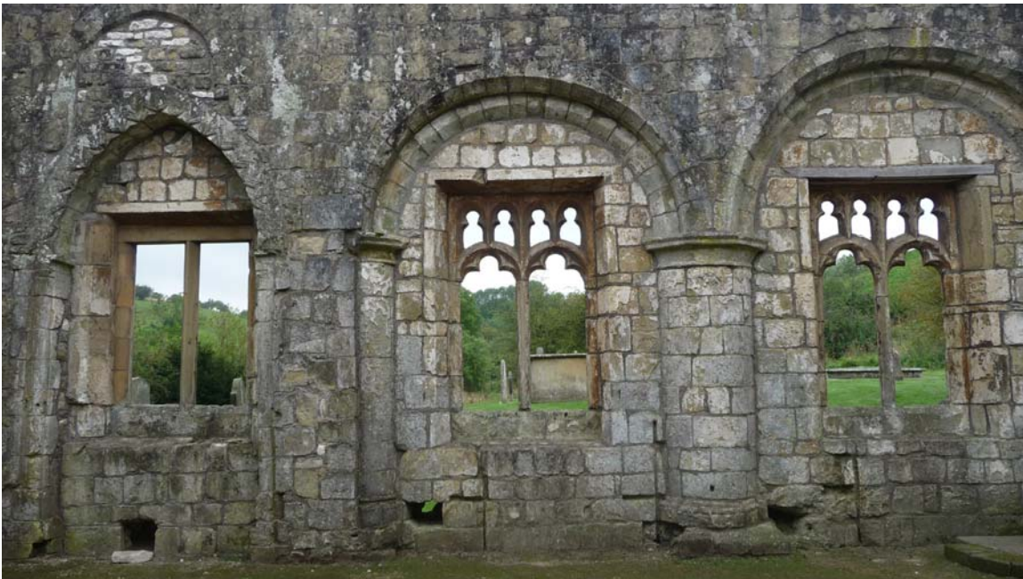
The church interior, showing the filled in pillars with two 16 th century windows. Notice to the left, top, a filled in circular window.
