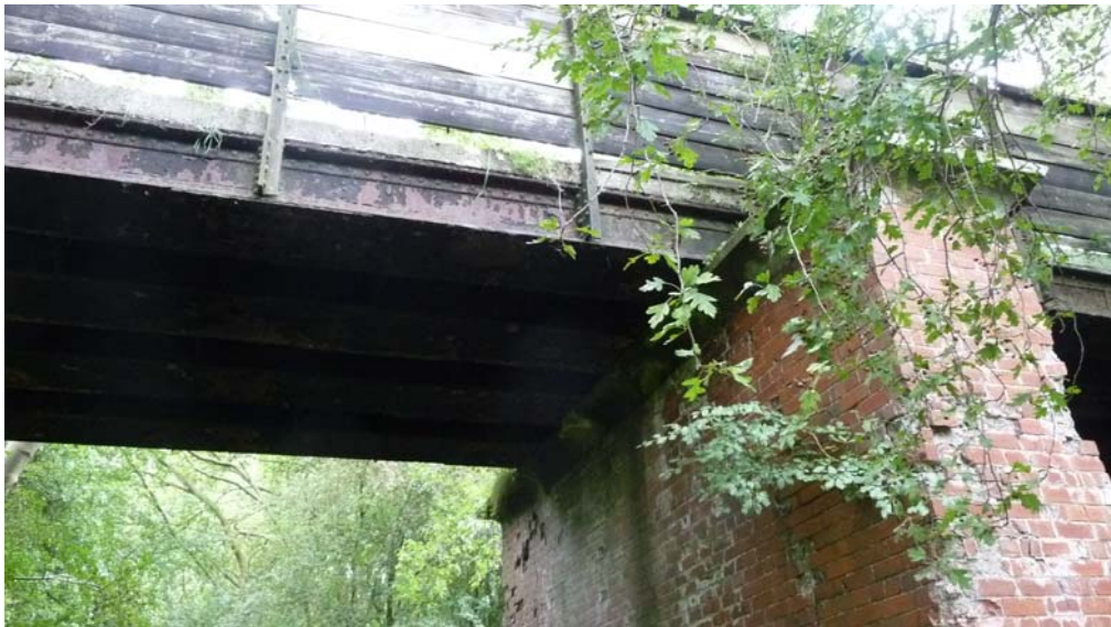
Detail of bridge support.
