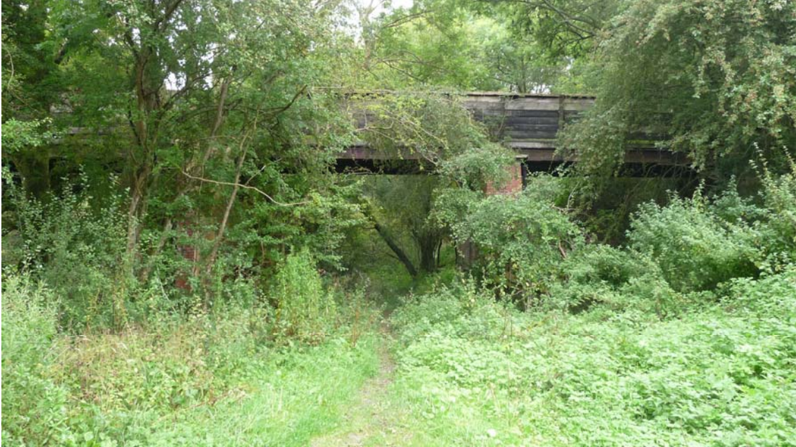
The foot-bridge, from the track-bed, looking towards the tunnel.
