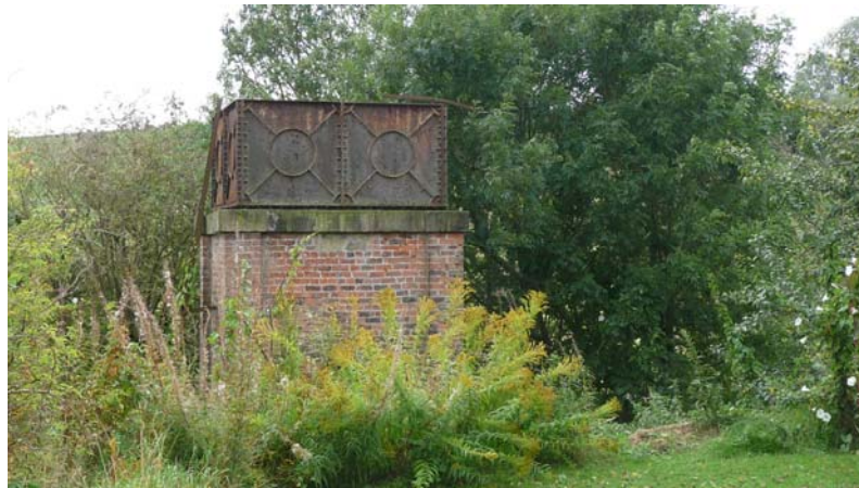
Water-tank at the station.
